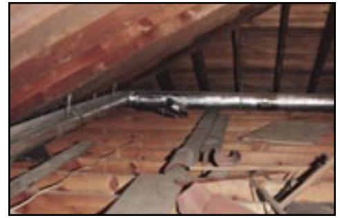
Unico's flexible ducts wind through existing construction, ensuring little to no remodeling is necessary for hvac installation.
