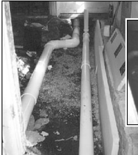
Using PVC, the lines for the Unico AC were constructed and buried 18" below grade.
