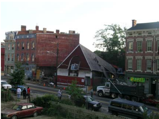
Threatened buildings in Cincinnati's Over-the-Rhine neighborhood.
