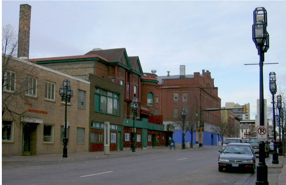
Historic commercial district in need of rehabilitation. Duluth, MN.
