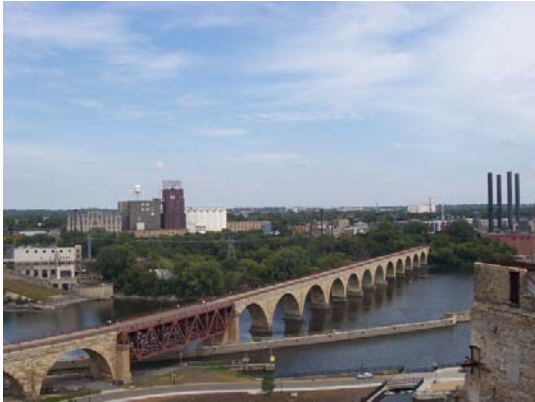
Pillsbury “A” Mill complex. Minneapolis, MN.
