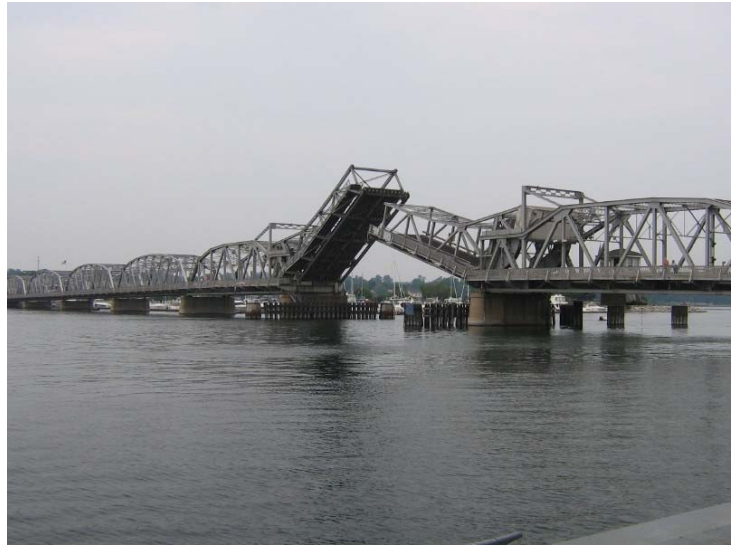
Michigan Street Bridge Sturgeon Bay, Door County, WI
