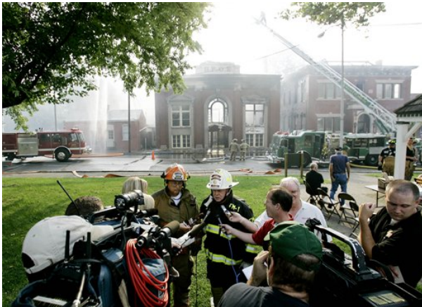
Fire damaged several buildings in the National Trust Landmark District in Madison, IN
