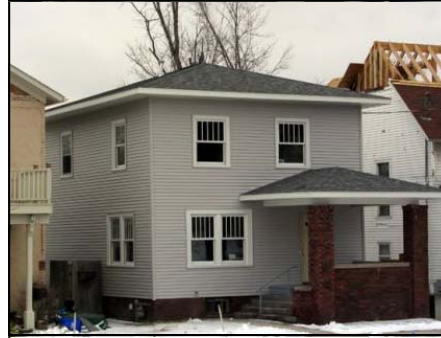
National Trust grants helped restore the front porch of 934 Iowa Avenue. The structure was considered for demolition but a new owner took great pride in restoring it. (Photo courtesy of City of Iowa City)
