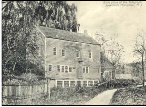
The Factory Building at Historic Speedwell Village in Morristown, NJ, seen in an 1888 postcard. This National Historic Landmark is the site of the first successful public demonstration of the electro-magnetic telegraph. A $325,000 grant will be used to address structural issues.
