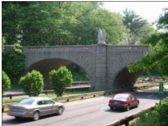
The Merritt Parkway Photo Courtesy of WMF
