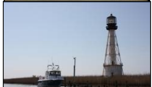
Port Eads Lighthouse in 2010, photo taken by FEMA
