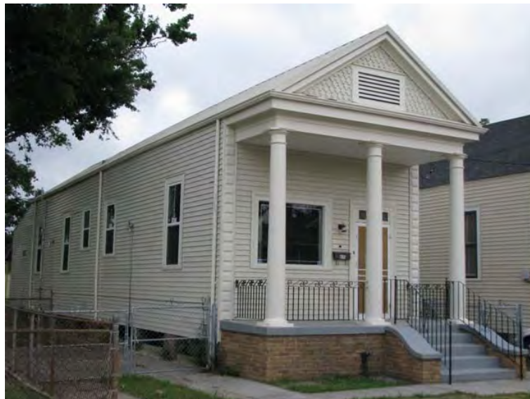
Photograph 1. 635 Angela Avenue, Old Arabi Historic District (April 26, 2009).
