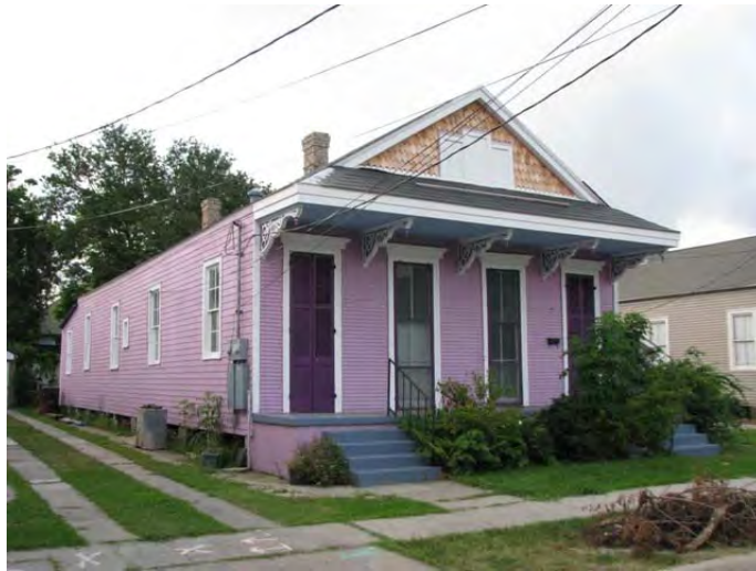
Photograph 1. 439-41 Angela Avenue, Old Arabi Historic District (April 26, 2009).
