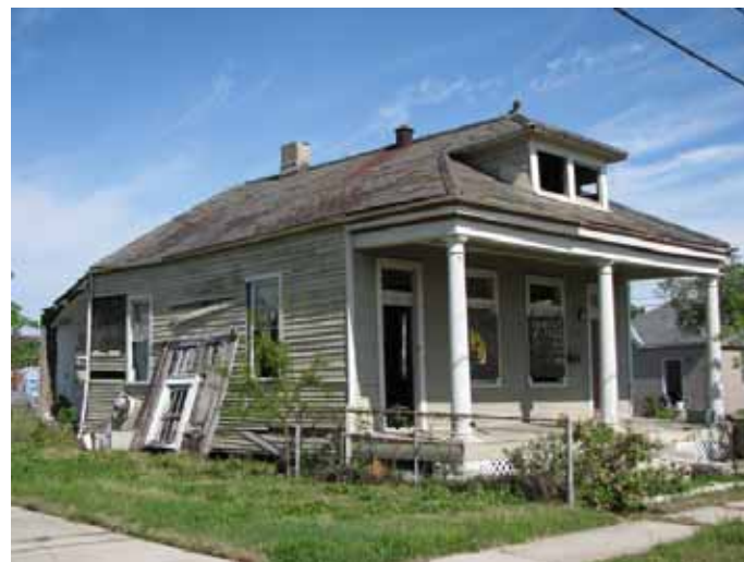
Photograph 1. 750 Angela Avenue, Old Arabi Historic District (March 30, 2009).
