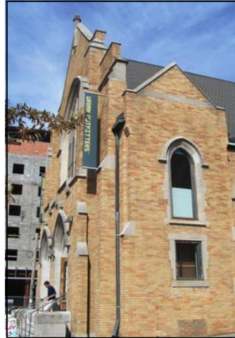
Cincinnati, OH — converted for Urban Outfitters retail store.
