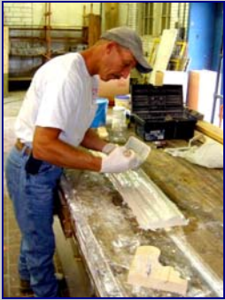
Photo: Durable Restoration 2008 - plaster restoration
