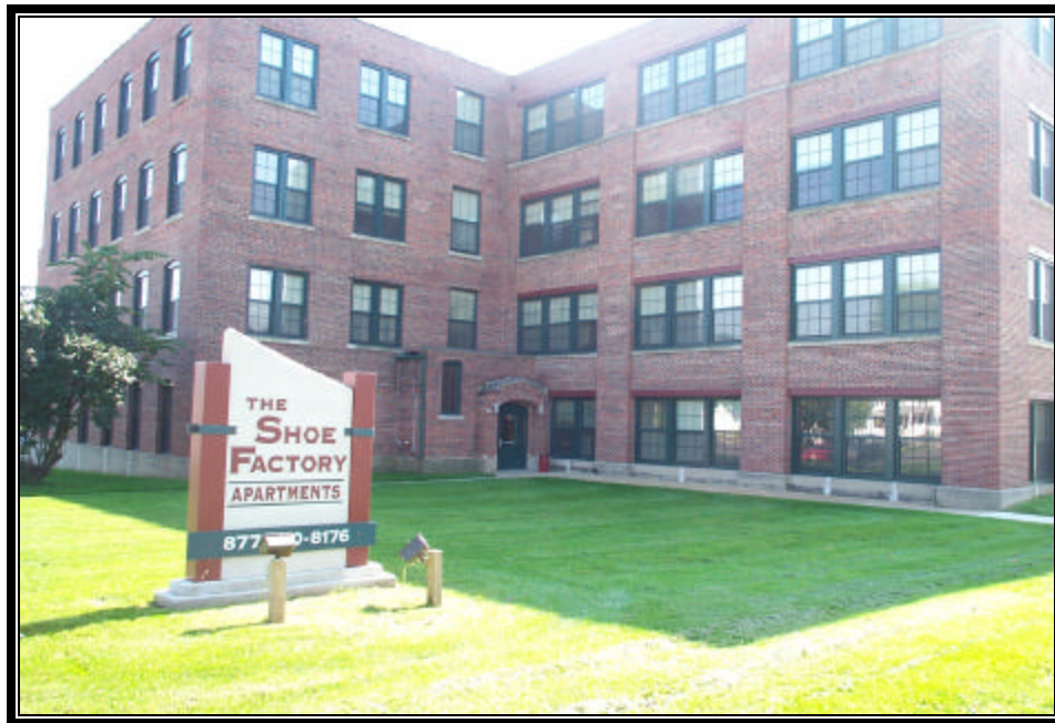
Smart Codes Rehabilitation Project in Beaver Dam, WI
