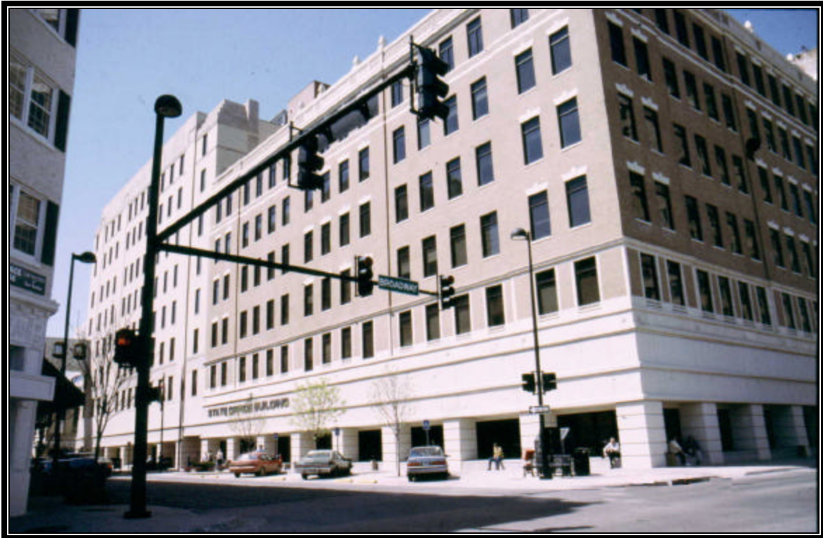
State Agency Building, Downtown Wichita, Kansas
