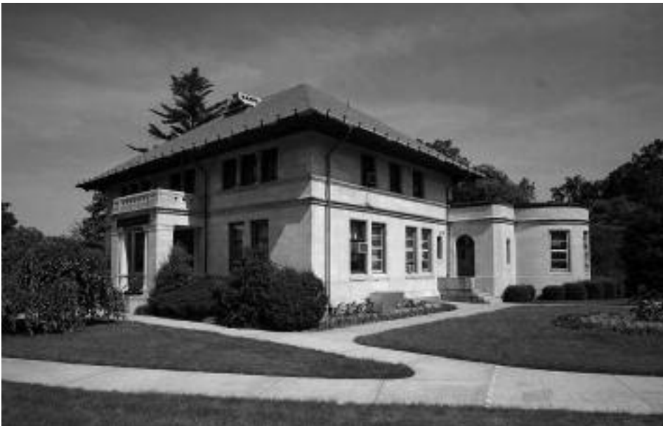
High LEED ratings can be achieved with historic buildings. With its rehabilitation of the President Lincoln's Cottage Visitor Education Center in Washington, D.C., the National Trust initially aimed for a silver rating but is now on track to earn gold. This project will also be used as a pilot to test the Alternate Compliance Path. Photo courtesy of the National Trust.
