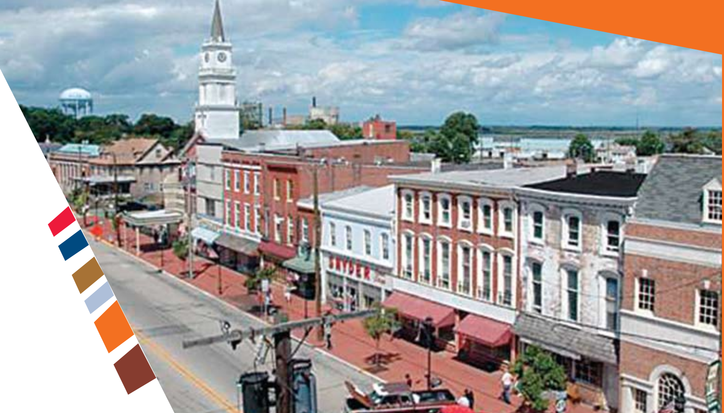
Downtown Salem, N.J., which is listed in the state, local, and national historic registers, possesses many architectural treasures.
