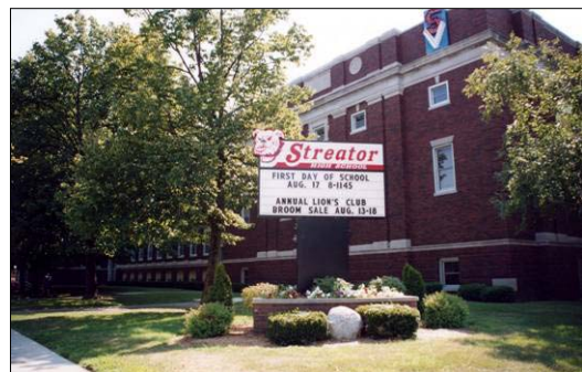
Streator High School, dating back to 1923, in Streator, IL. [LPCI]
