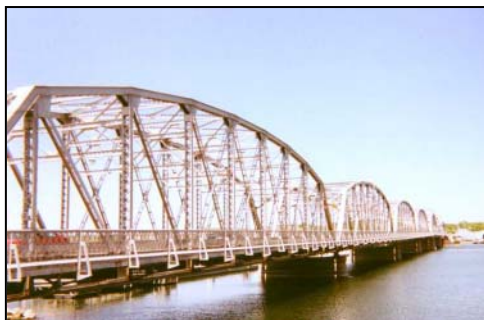
The Michigan Street Bridge in Sturgeon Bay, Wisconsin [NTHP].
