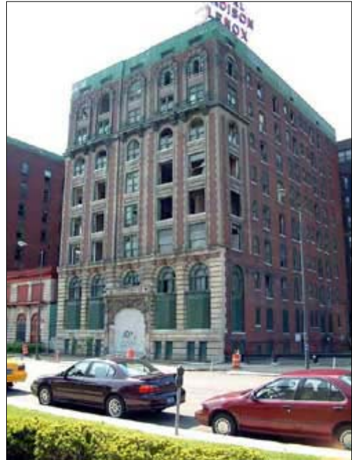
The Madison-Lenox, a three-building complex – including the 8-story Madison, built in 1900; an adjacent two-story restaurant; and the Lenox, built in 1903 – was demolished in June.
