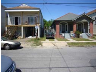
Some federal funding programs have provided recovery assistance that has required even historic structures to be raised eight to ten feet up in the air. [NTHP]
