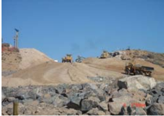
View of the cut through the West Mesa escarpment. [Rocky Archuleta]
