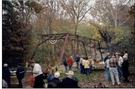
The LDF has worked closely with state and local preservationists to save the historic Wilson Bridge in Carroll County, IN. [NTHP]
