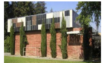
IBM Building 25 in San Jose is a 1957 International-style building where the "flying head disk drive" was invented. [Preservation Action Council of San Jose]
