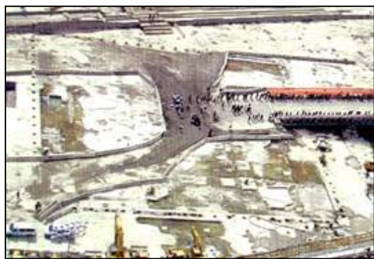
The bases of the box-beam columns outlining the twin towers are still visible at the World Trade Center site [Courtesy of the Coalition of 9/11 Families].
