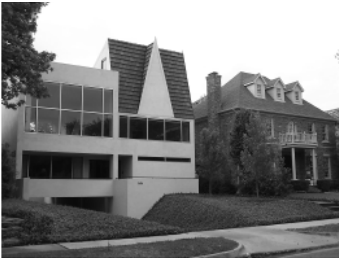
Without tools to manage teardowns, the overall character and charm of a historic neighborhood begins to disappear, replaced by a hodgepodge of “McMansions” and forlorn-looking older homes. Photo by Adrian Scott Fine.
