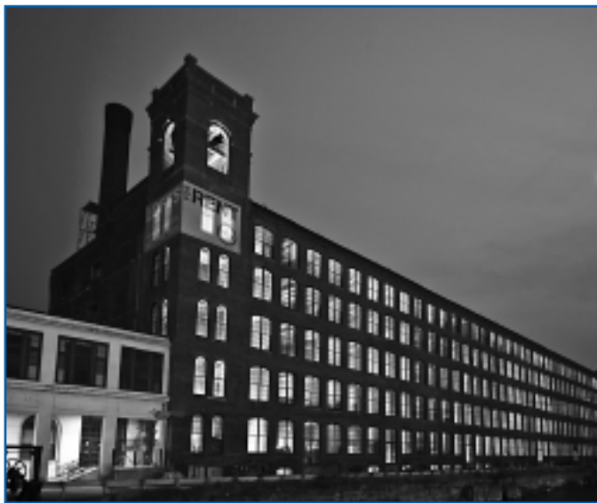
The Washington Mill project brought over $40 million of investment and 155 permanent households to a struggling Massachusetts community. Photos courtesy of the Architectural Heritage Foundation.
