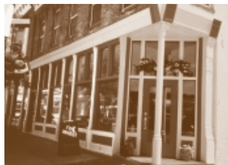
After suffering severe flood damage, many main street property owners in Darlington, Wis., retrofitted their buildings by constructing a new first floor above the 100-year flood plain level.
