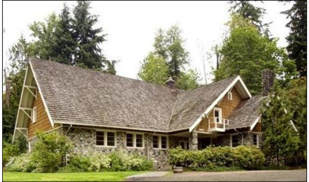
Preston Community Clubhouse, Preston
